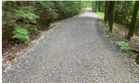
Hemlock Place – after – Left photo from midpoint on the road looking downhill, road resurfaced with Bluestone gravel. Right photo looking uphill at replaced culvert with stabilized outfall and improved ditching.
