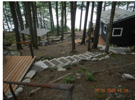
Infiltration steps - Harriman Pond
