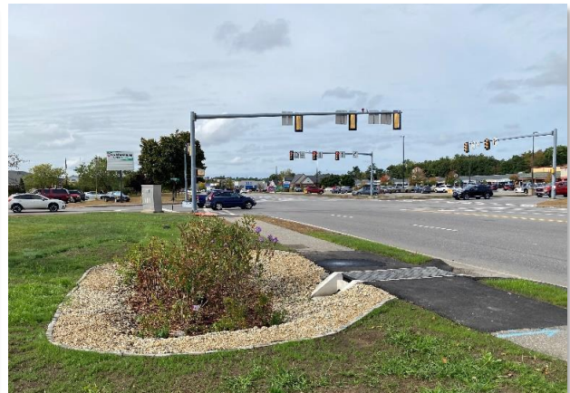
Completed bioinfiltration system with native plantings.
