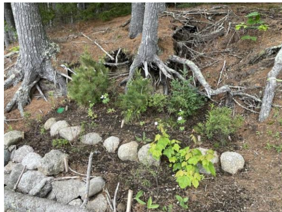
Shoreline stabilization using living shoreline concepts – limiting the use of stone, and combining with coir logs and native plantings
