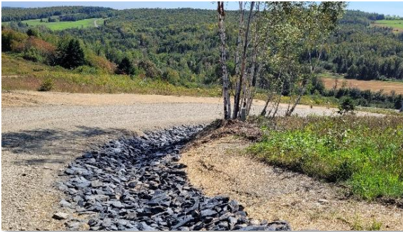
Rock lined ditch and regrading on Black Lake Road, Ft. Kent
