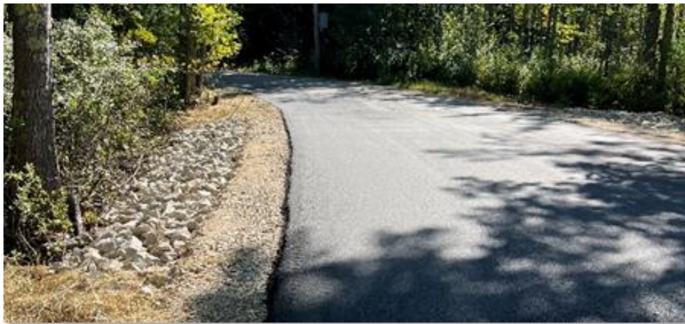
A "rock sandwich" restores hydraulic connectivity of a wetland, and prevents repeated overtopping on Poor Farm Rd., Lyman
