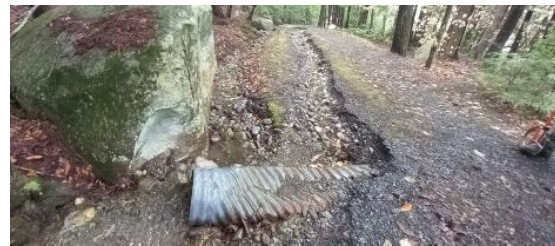
Hemlock Place -before – Left photo from midpoint on the road looking downhill at erosion caused by failed culvert (right photo). Right photo looking uphill at failed culvert.
