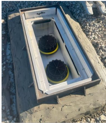
Fabco StormBasin insert with two filter cartridges will filter bacteria in runoff. Runoff once filtered will infiltrate through the enhanced drywell
