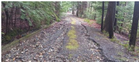
Hemlock Place -before – Left photo from midpoint on the road looking downhill at erosion caused by failed culvert (right photo). Right photo looking uphill at failed culvert.
