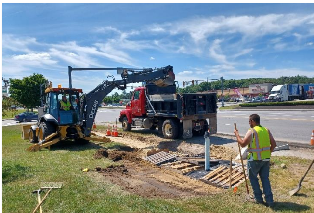
Installation of bioinfiltration system to treat polluted road runoff.
