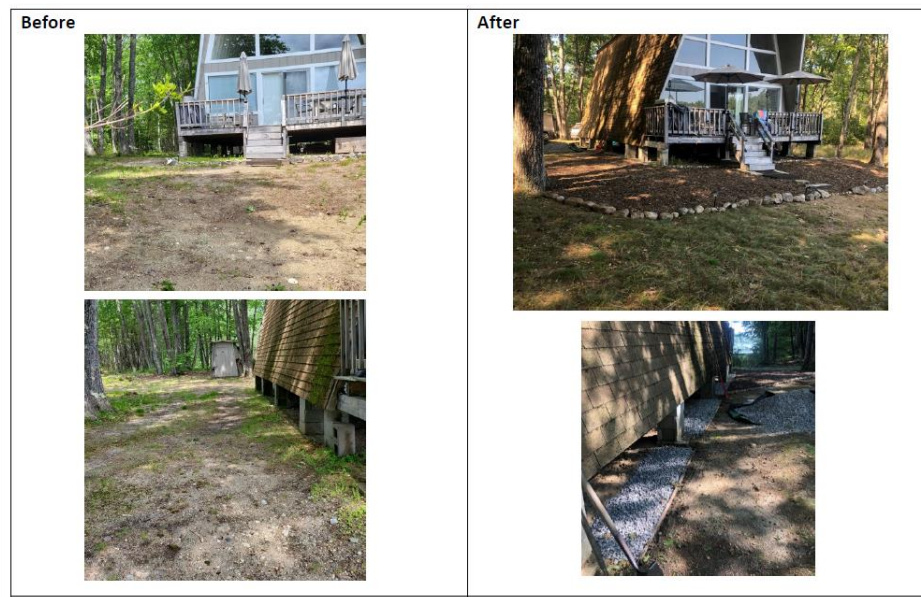
Before and After photos from a residential matching grant project which included a dripline trench and erosion control mulch
