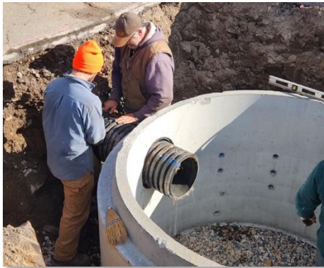
Installation of an enhanced drywell that allows stormwater to infiltrate through crushed stone.
