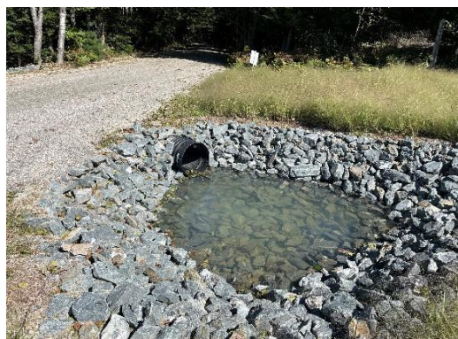
Dirt camp road BMP - Cross drain culvert plunge pool
