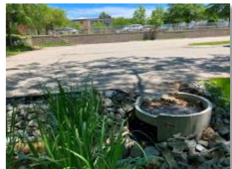
Biofiltration BMP at the Brown Elementary School
