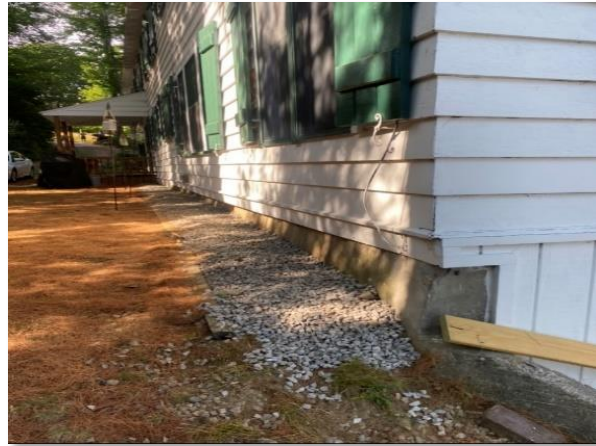
Infiltration trench at lake side camp
