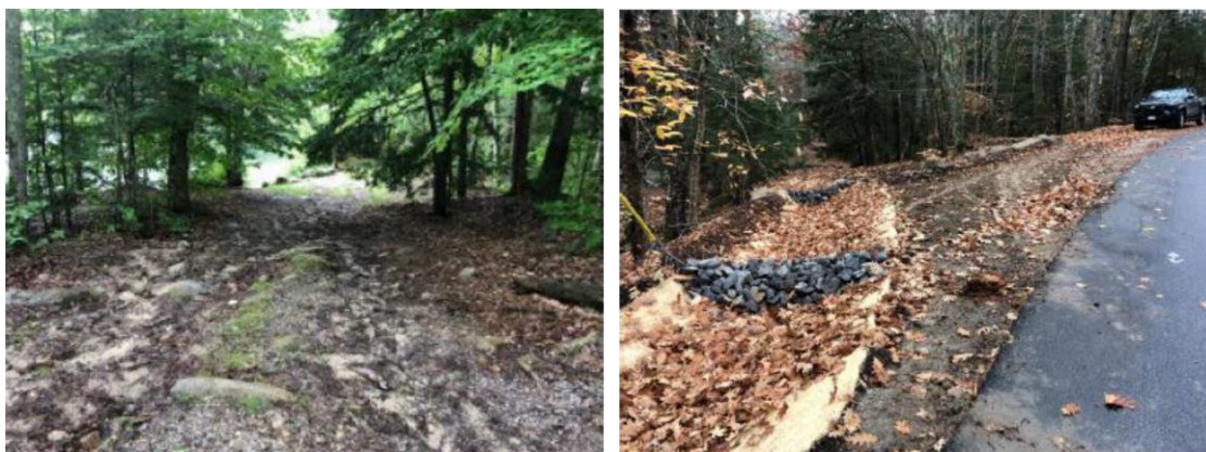
Left photo – “before” condition looking uphill from the boat launch to the road. Right photo – “after” condition at the top of the hill showing newly installed ditch and turnout with check dams.
