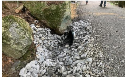
Hemlock Place – after – Left photo from midpoint on the road looking downhill, road resurfaced with Bluestone gravel. Right photo looking uphill at replaced culvert with stabilized outfall and improved ditching.
