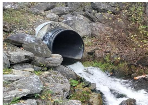
Perched Culvert on McHugh Brook
