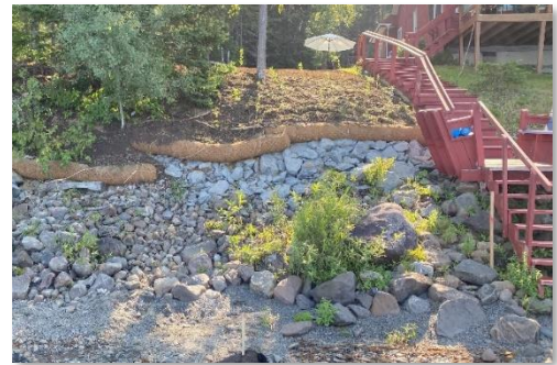
Shoreline stabilization on Cross Lake
